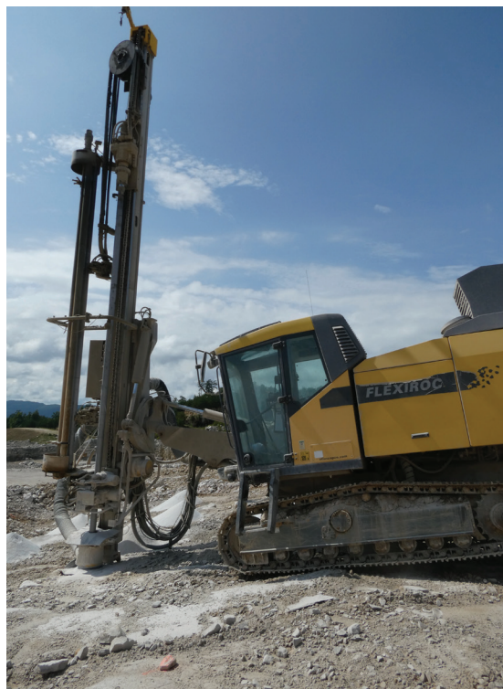
Fig. 4 Drilling silica, Silica Mountain. Photo: Erin E. O'Connor.
